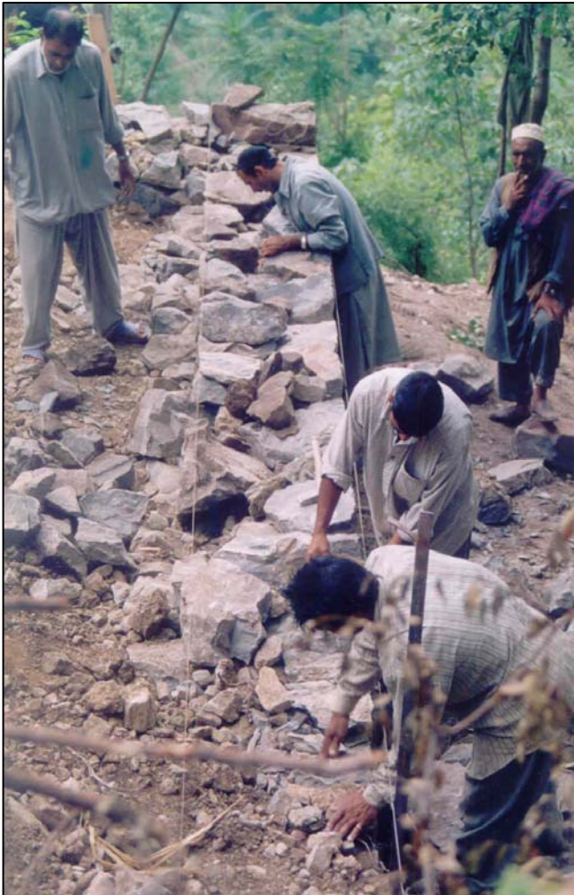
Learning the use of steel rods in place of through stones
